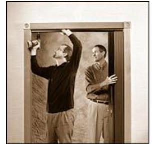
Transfer the door to the attached end of the track. Finish attaching the track with 1 1/2" #8 Pan Head screws.
